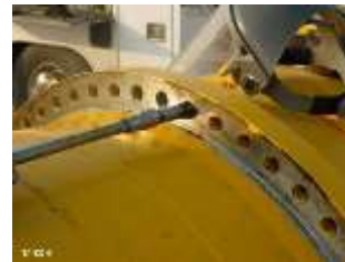
Cleaning paint and rust prior to torquing
