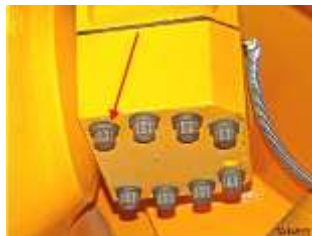
Arrow indicates location to be cleaned
